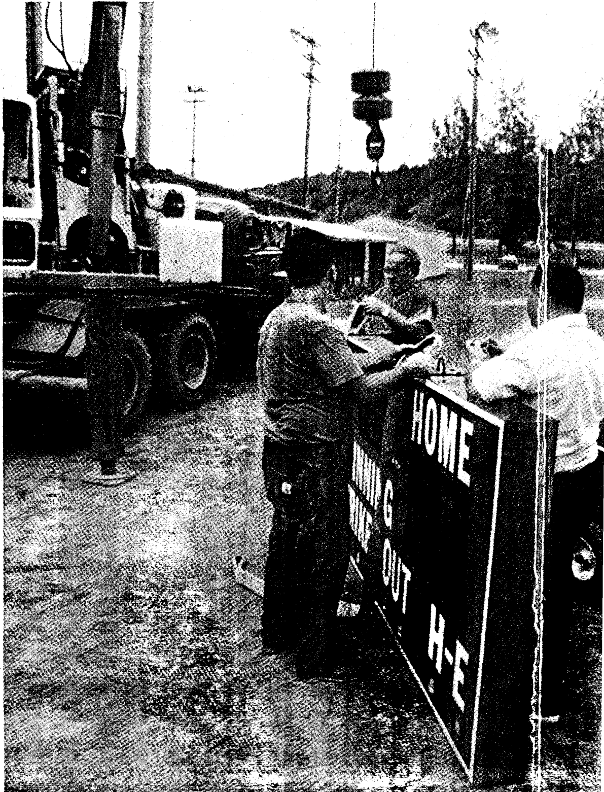
LYNN NICKLES OF NICKLES CRANE Service secures one of the scoreboards for hoisting with help from Dick Davis and Jim Parris (right) Friday afternoon at Miller Fields in Wooster. All three Wooster Youth Baseball fields are getting electronic scoreboards.
